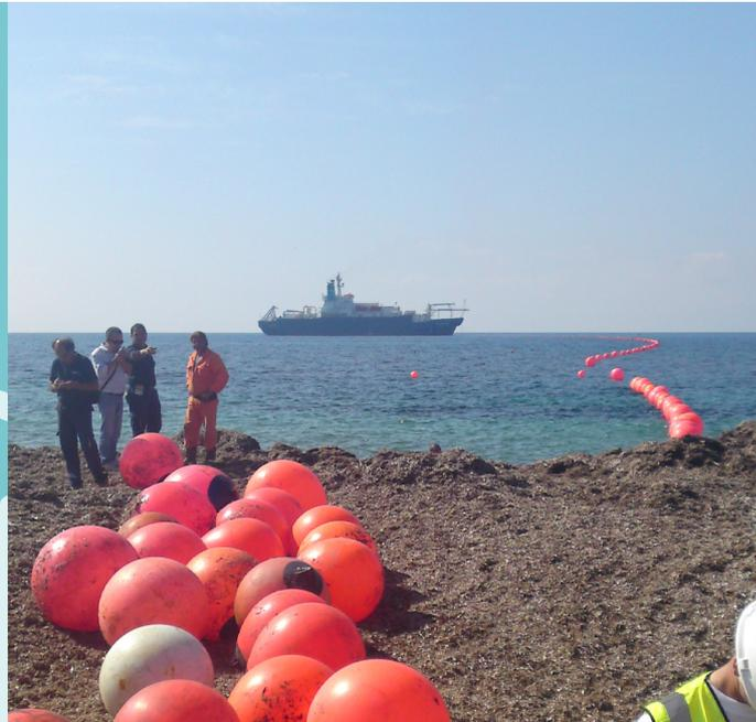
Tunisie Telecom contracted (Huawei Marine Networks) HMN and Global Marine Systems Limited for the supply and installation of fibre optic cable for the Hannibal submarine cable system between beach manholes in Kelibia, Tunisia and Mazara del Vallo, Sicily. The 177.5 kilometres of submarine cable was provided by Nexans, and loaded at the port of Rognan, Norway.
